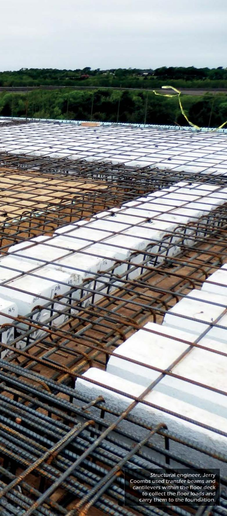
Structural engineer, Jerry Coombs used transfer beams and cantilevers within the floor deck to collect the floor loads and carry them to the foundation.
