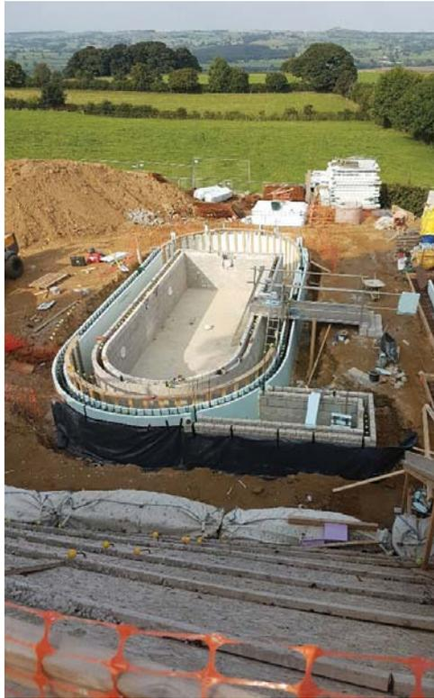
Figure 2a and b (above and below): The basement level needs to withstand lateral pressures and meet waterproofing standards to BS 8102.
