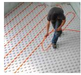
NUDURA has brought innovation to the market with our line of Insulated Concrete Forms, that innovation continues with HydroFoam™. Installation is fast and easy compared to traditional foam insulation which requires multiple steps to run radiant heat piping. The 4' × 4' (1.2 m × 1.2 m) boards, available in two thickness, are easily installed with an overlapping interlock on all four sides, ensuring the boards are locked in
